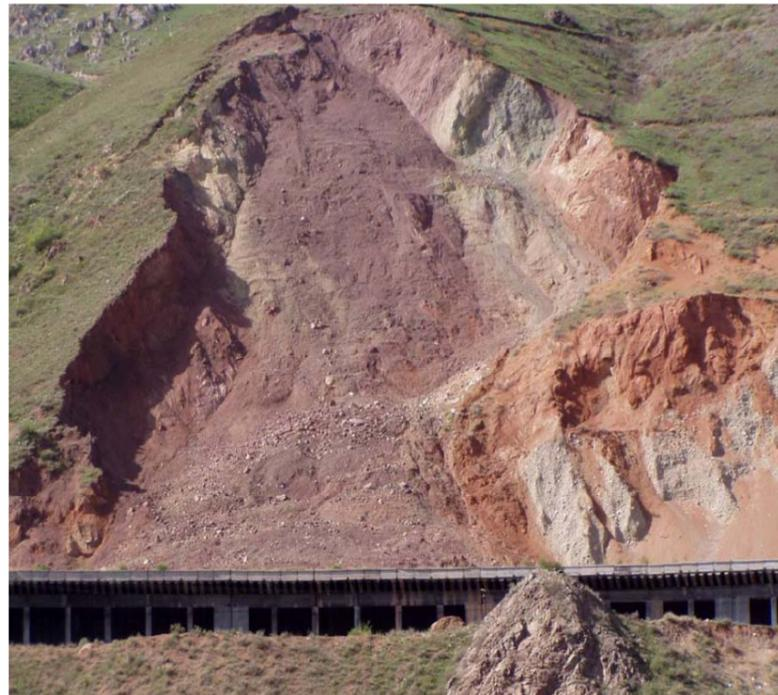
Fig. 34. Landslide above the railway gallery on the 115-th km of the Bishkek – Balykchi road in Boom canyon (photo made by S.A.Erochin). This active landslide threatens to destroy the gallery. They regularly clear off the blocks moving down to the gallery.
