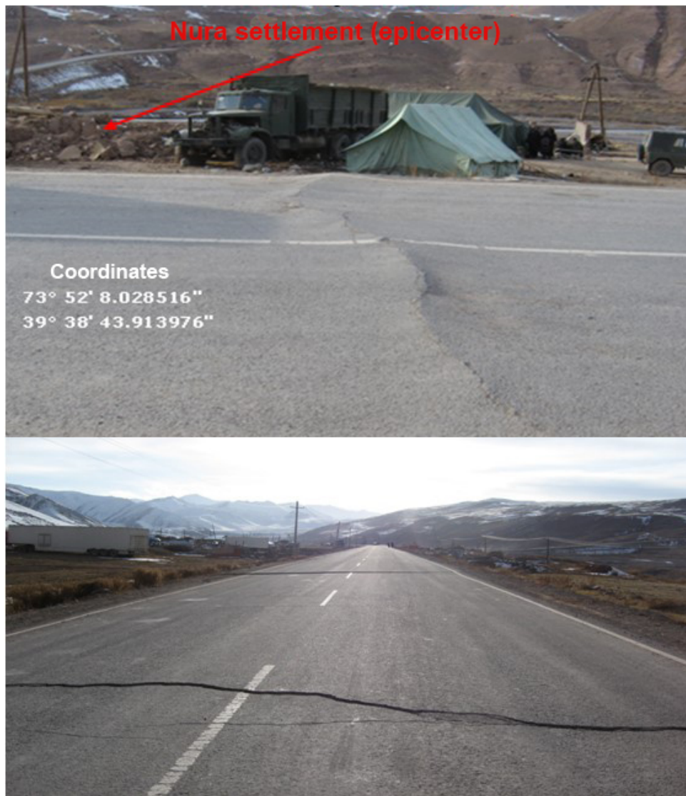
Figure 1.4.2. Cracks (lower part of photo) and “waves of deformation” (upper part) were observed in the vicinity of Nura settlement at distances up to 2-3 km (photo taken by Meleshko A.V.)
