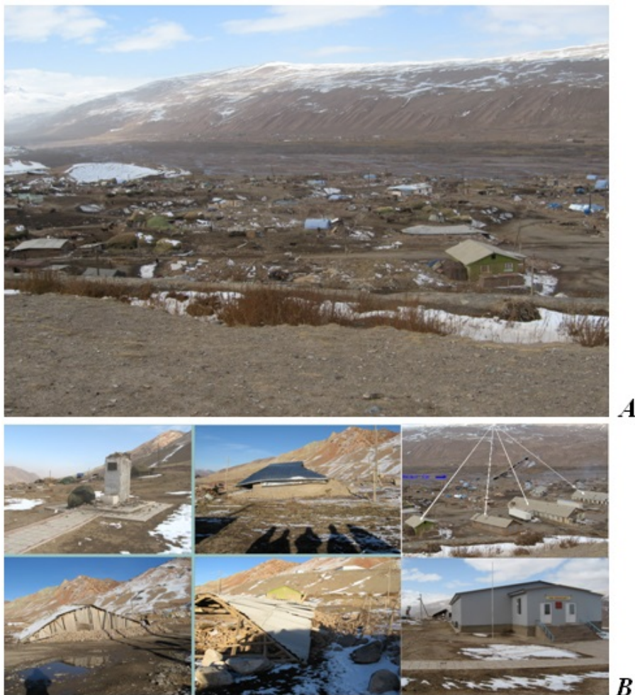
Figure 1.4.1. Nura village after the earthquake (A), typical structural damages (B) (photo taken by Meleshko A.V.)
